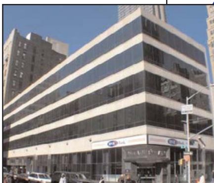
855 Avenue of the Americas - Bernstein Family multi-tenanted and fully occupied office building.
