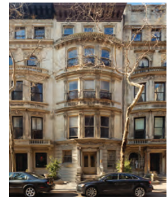
18 West 76th Street Manhattan, NY $11.7 MILLION Multifamily
