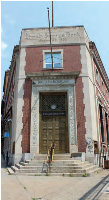
525 Broadway Brooklyn, NY $32.8 MILLION Development Site
