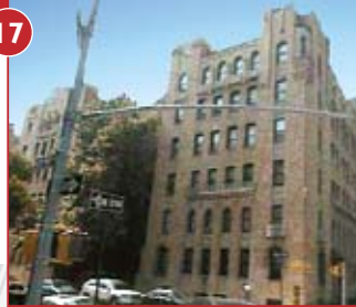
750 PELHAM PARKWAY SOUTH
