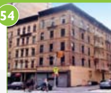
70-74 EAST END AVENUE
