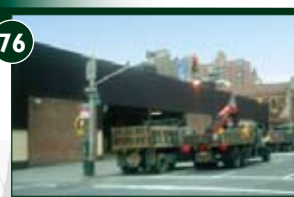
169 TENTH AVENUE (AKA 502 WEST 21 ST STREET)
