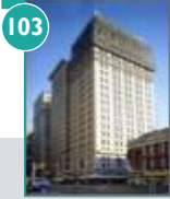
103 201 PARK AVENUE SOUTH
