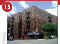
441-449 MORRIS PARK AVENUE (1185 LEBANON STREET)
