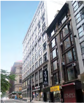
4 and 6 West 37th Street Manhattan, NY $20,000,000 Development Site
