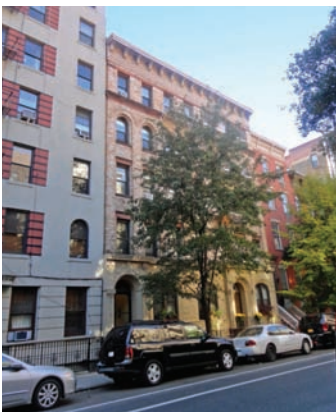
222-224 West 21st Street Manhattan, NY $16,750,000 Multifamily
