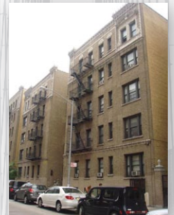
712 West 176th Street New York, NY Sold: $5,350,000 Apartment Building
