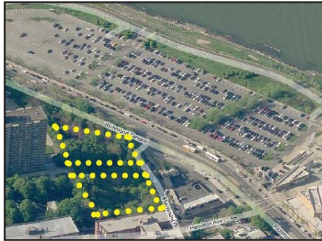
$33,626,000 Non-Performing Loan Liberty Towers & Waterfront Commons Staten Island, NY
